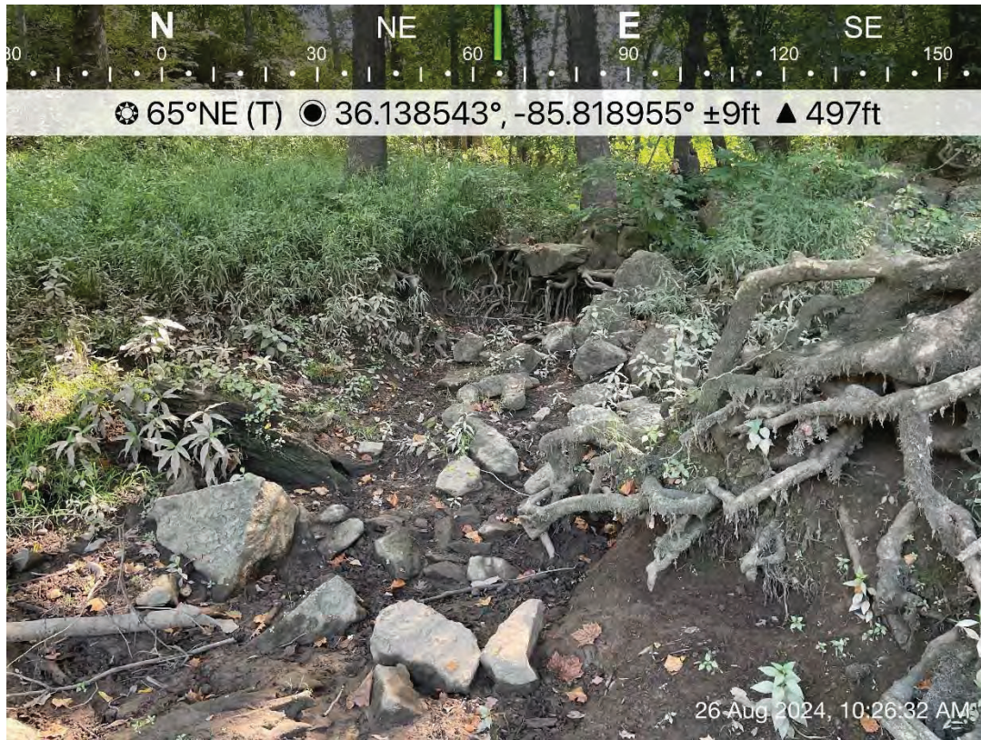
Photo 3. WWC-1 looking up gradient at scoured area shortly after concrete lined portion ends
